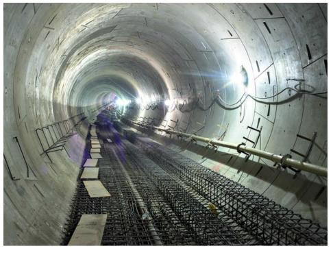
Reinforcing steel and concrete will be placed in bottom of tunnel to form trackbed and benchwalls
