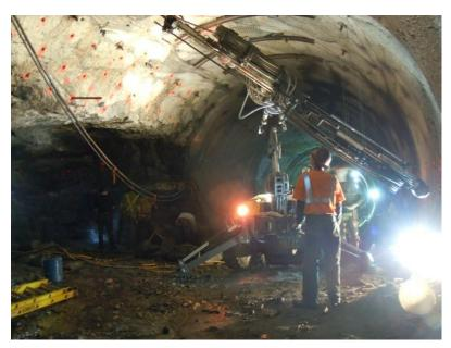
Cross passages between tunnel tubes will be excavated through controlled drilling and blasting (2 weeks per cross passage)
